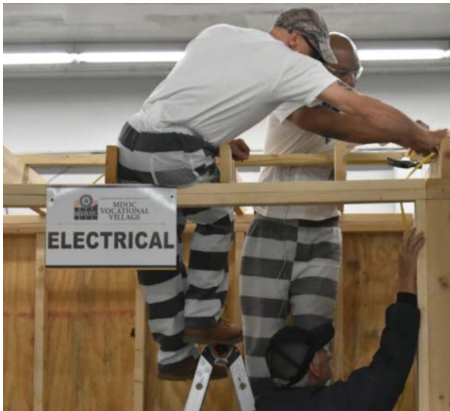
Participating inmates in the Vocational Village at the Central Mississippi Correctional Facility put their electrical wiring skills to use with practice on demonstration structures.
